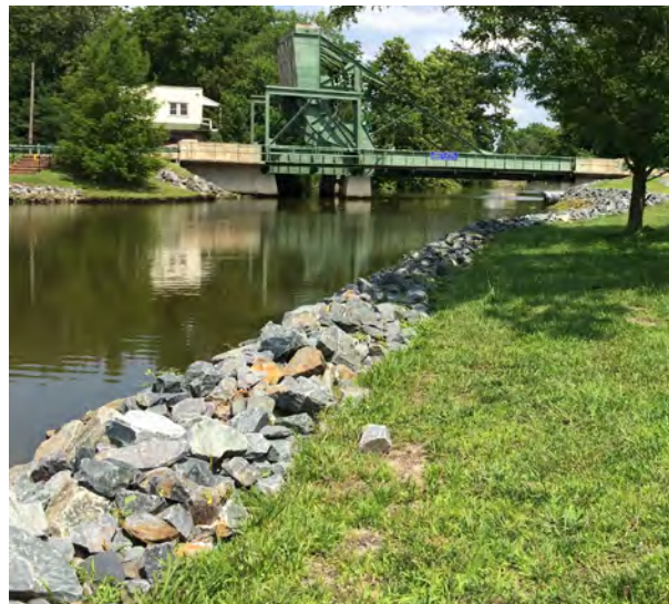
rip rap stone shoreline conditions
