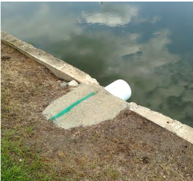
SD1-P1 outfall along north bank of Broad Creek
